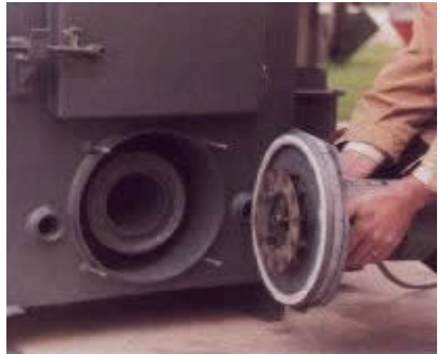
Figure 27: Direct-drive fan removed from boiler exposing the heat exchanger.
